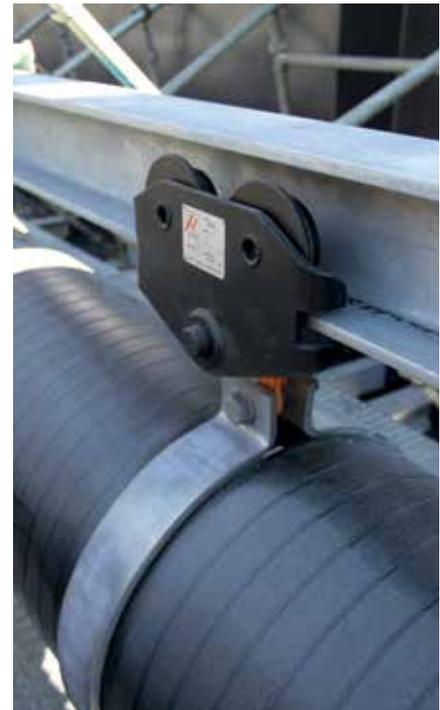
Sveros blockvagnar brukas inte bara inom industri - här har man använt sig av vagnarna vid montage av fjärrvärme och fjärrkyla under brobygge. Svero trolley is not used only in industry - this has been used by coaches during installation of heating and cooling during the bridge construction.
